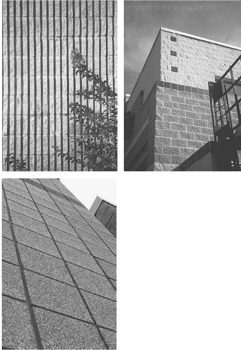
Figure 4-11 Ribbed, split-face, and burnished concrete block.
